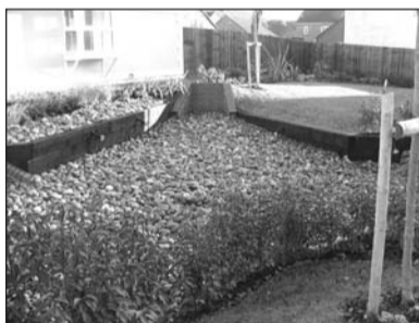
A pond at the Hermitage development linked to the SUDS system
