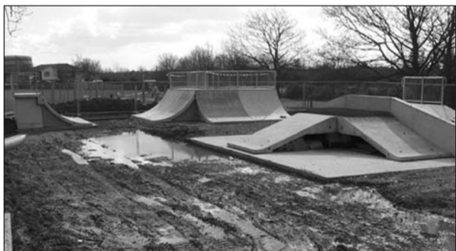
Emsworth Skatepark nearing completion 10 March
