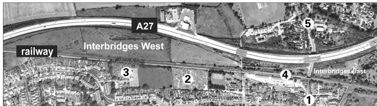
Interbridges East and West industrial sites
