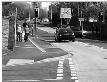
Shared pedestrian cycle path awaiting signs
