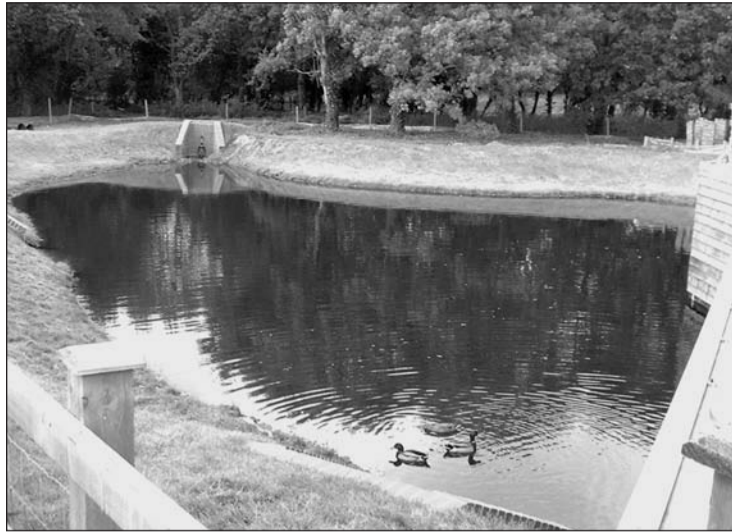
Balancing pond showing the two oak trees under threat, centre back.
